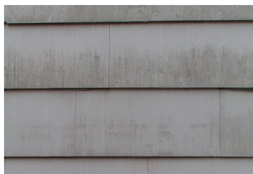
Exterior wall siding
