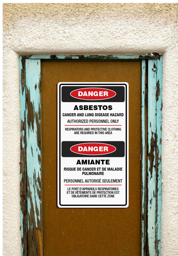
Warning sign for a Type 2 asbestos work entry requirement outside of a mechanical space containing ACM.
