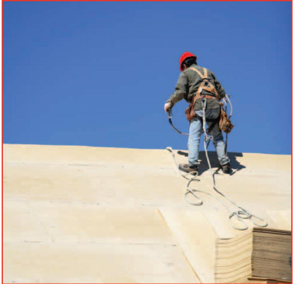
*Using fall protection systems like guardrails, fall arrests and safety nets when doing residential construction is critical to saving lives.*
